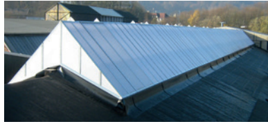
Saddle rooflight after refurbishment
