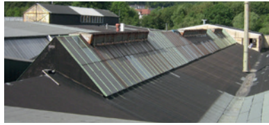
Wired glass saddle rooflight before refurbishment
