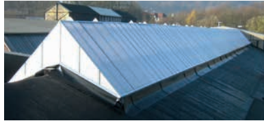
Saddle rooflight after refurbishment
