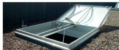
JET VARIO light flap with SHEV device and electrical motor after SHEV release in the final position
